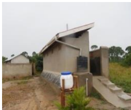
ECOSAN LATRINE AND STALL
